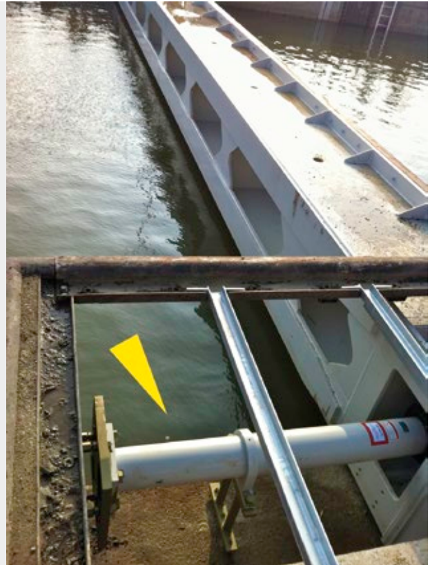
Heavy safety shock absorbers, which are specially designed for this application, are able to brake in lock masses of up to four million kg Mourik Limburg BV, 6101 AJ Echt, Netherlands
